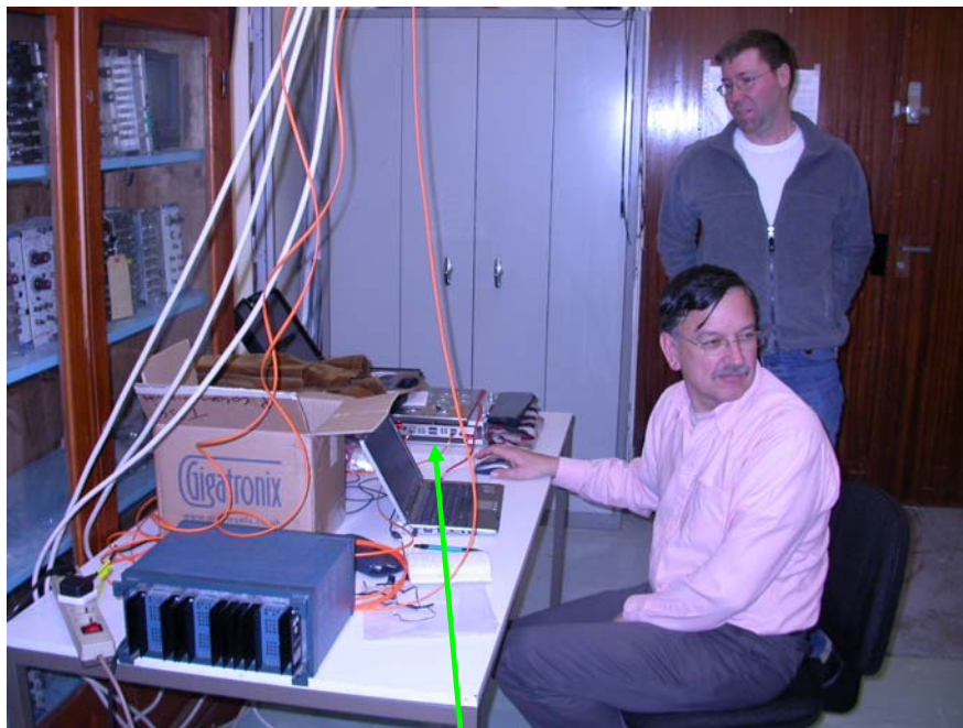
Water cooled digitiser Core module with control laptop, Orange fibre optic links, and white analogue Camera link cables.
